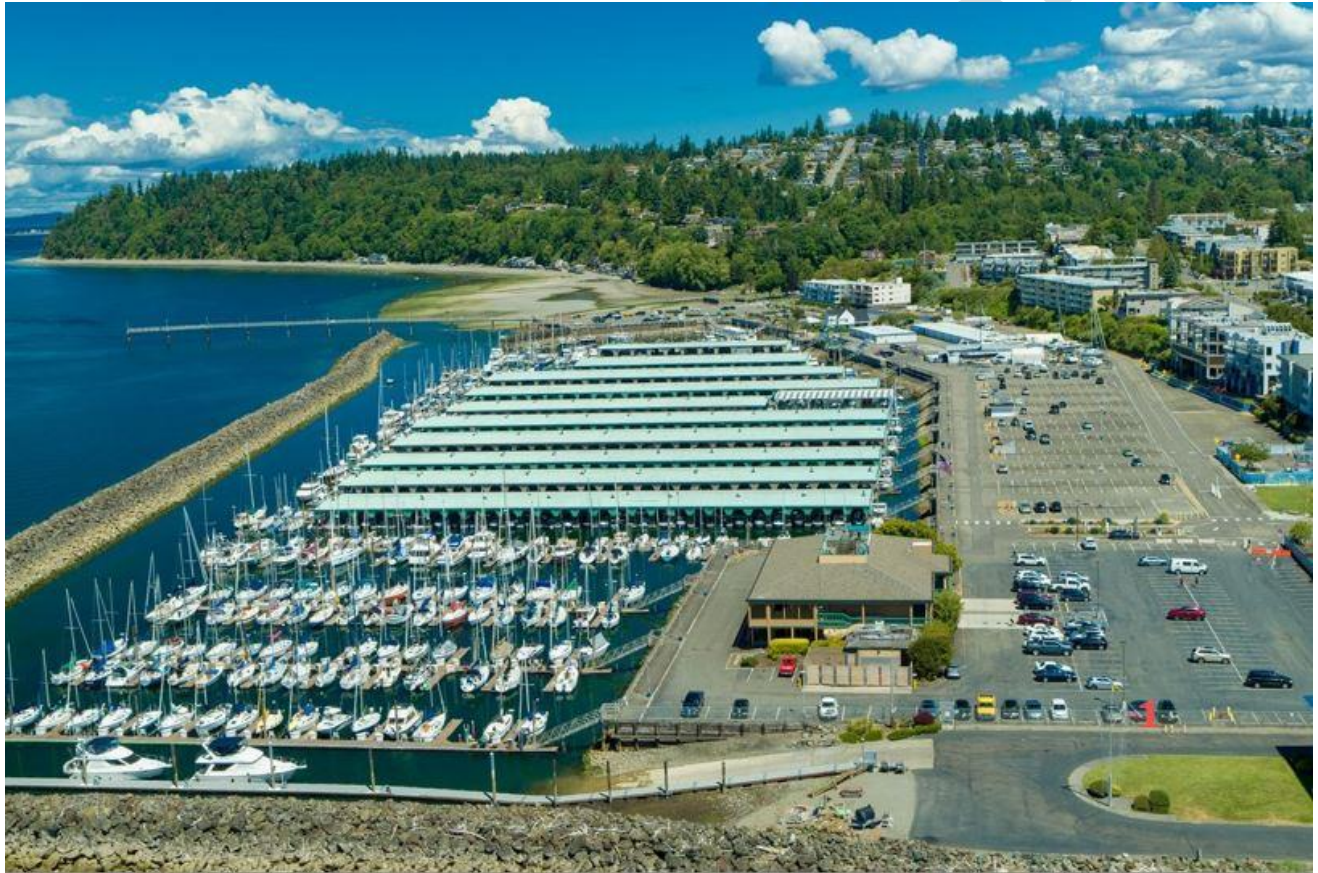
Figure 1. City of Des Moines Marina
