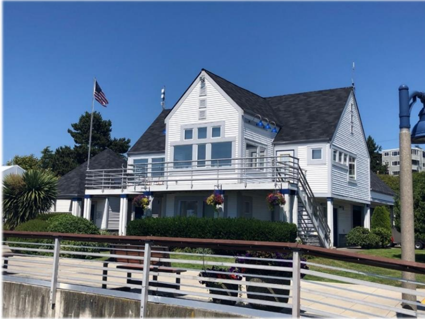
Figure 5-1. Marina Office Building July 2021
