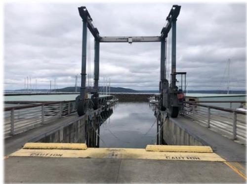
Figure 2-9. Travel Lift Pier
