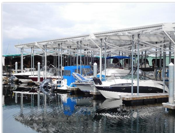
Figure 4-2. Covered Moorage on J-Dock
