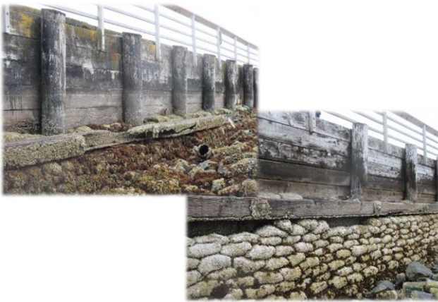
Figure 2-13. Old North & West Timber Pile Bulkhead
